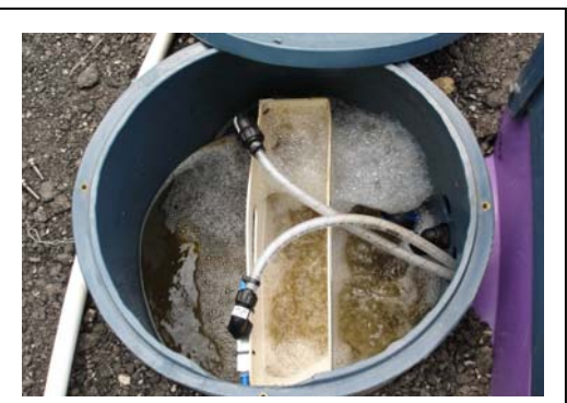
廁所水淨化過程 Black water Bio-treatment
